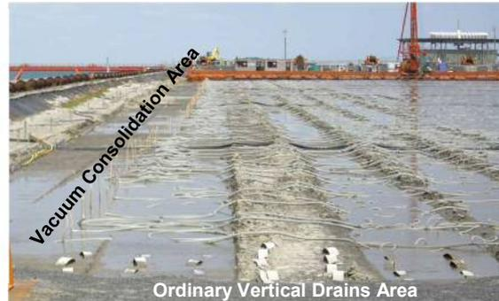
Photo 1. Ground surface condition installed vertical drains by PDF-system
