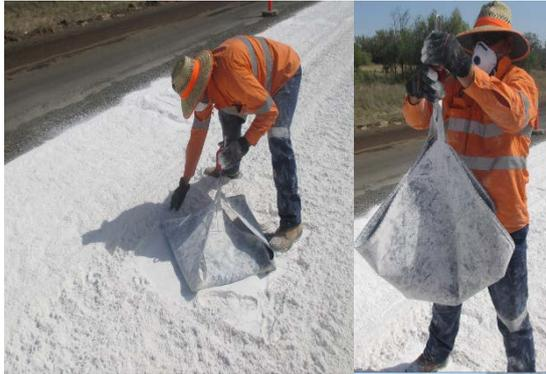
Fig.4 Matt Test carried out on site
