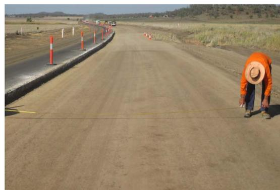
Fig.3 Boxed-out section for lime stabilising
