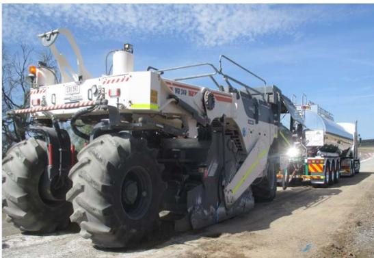
Fig.8 Foam bitumen stabilizing work
