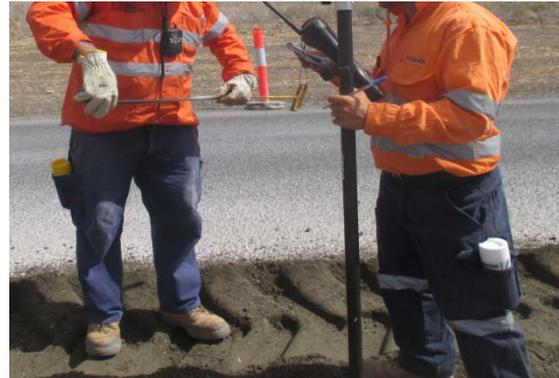
Fig.6 Depth control (manual measurement using trimble)
