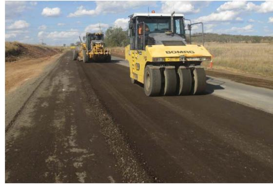
Fig.9 Foam bitumen stabilising work
