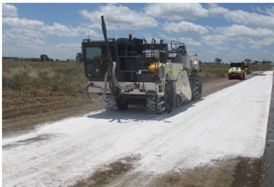
Fig.5 Subgrade lime stabilising works (Dry run)
