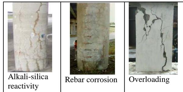
Fig.1 modes of RC columns failure [1]-[2]
