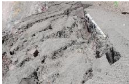
Fig. 15 Toppling failure mechanism at W22 wall of the west slope within the Magazine Shale domain at ramp level 3400, looking south of the pit.
