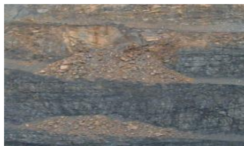
Fig. 17 Wedge failure at W21 wall at ramp level 3376, looking west.
