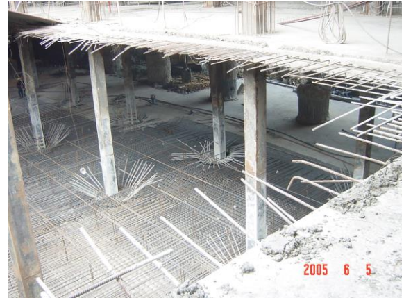
Fig. 10 Basement construction during excavation to the final depth
