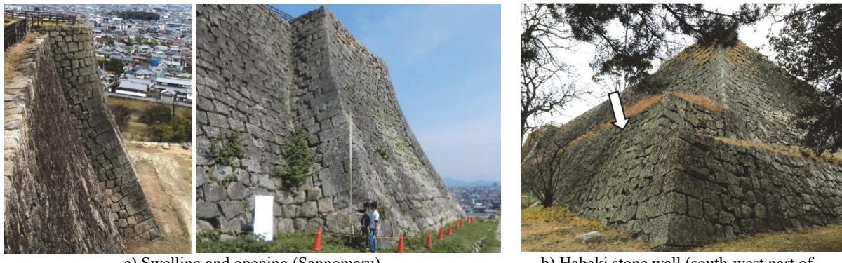
Fig. 2 Typical deformed stone wall a) and Habaki stone wall b)
