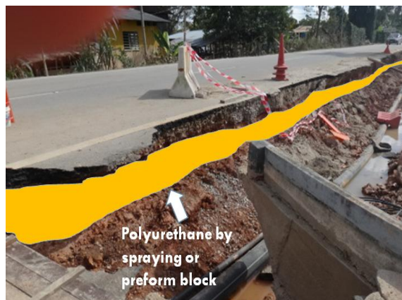
Fig. 1: Polyurethane layer by spraying or preformed block
