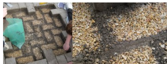
Fig. 2. Sediment Accumulation Pattern on Bedding Aggregate [2]
