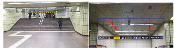
Fig.8 Inspection of structure interface status in situ
