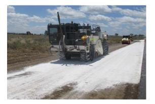
Fig.5 Subgrade lime stabilising works (Dry run)
