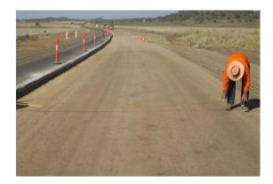
Fig.3 Boxed-out section for lime stabilising
