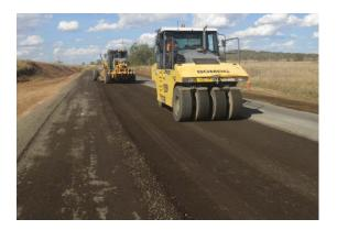
Fig.9 Foam bitumen stabilising work
