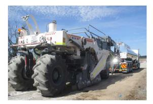
Fig.8 Foam bitumen stabilizing work
