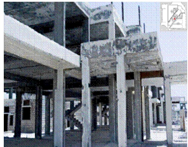
Fig. 3. Dilapidation photo in area TA1.
