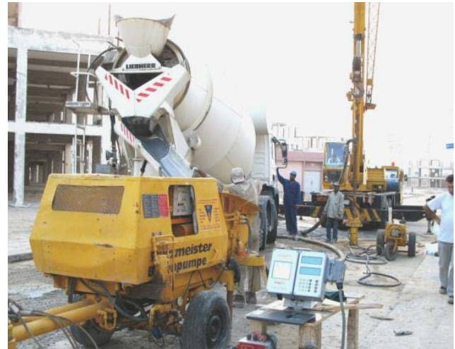
Fig. 2. Delivery and pumping of cavity filling mortar.
