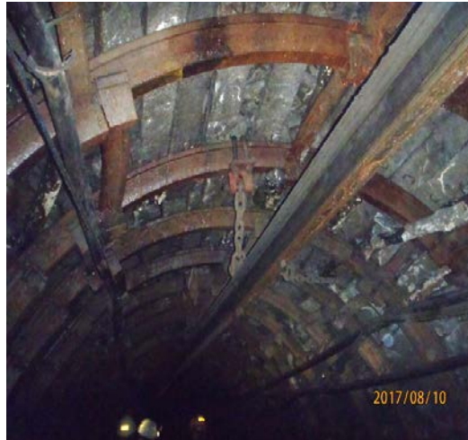
Fig. 3 The outline of the roadway with traditional support
