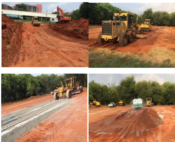
Fig.12 Compacted ground with and without cement stabilization
