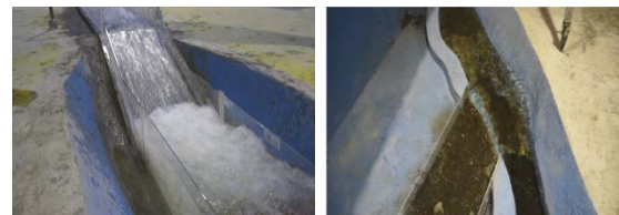
Fig.12. The flow condition of the stilling basin and outlet channel
