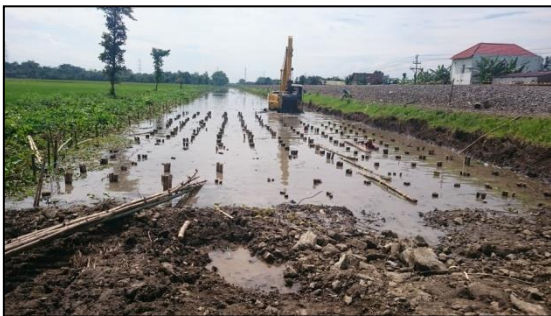
Fig 5. Driving bamboo piles [14]
