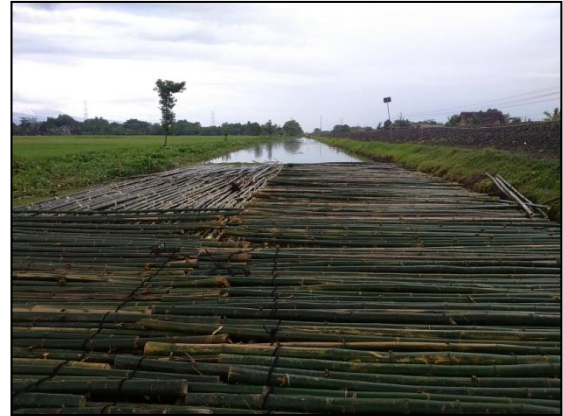
Fig 6. Installation of bamboo mattresses [14]
