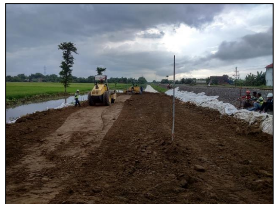
Fig 7. Spreading the fill material and compaction [14]
