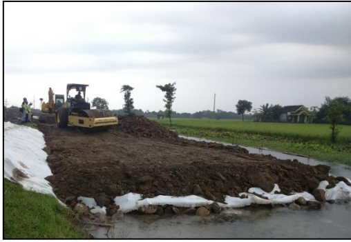
Fig 8. The Geosynthetic reinforcement applied [14]
