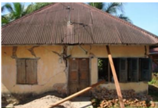
Fig.6 Damaged house due to Padang earthquake
