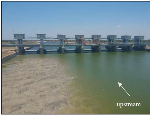
Fig. 5 Sediment deposition after Sembayat Weir construction (on 20 September 2019)
