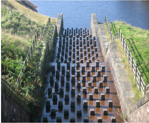
Fig. 2 Baffled spillway with concrete block baffles located at Yeoman Hey Reservoir, Saddleworth, UK. One concept presented in this paper would be to have biochar encased in heavy duty wire mesh boxes, forming anchored baffle elements, replaceable using light crane. Research needs to be carried out to optimise geometrical specifications, in relation to performance versus economic considerations.
