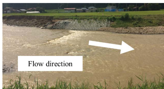
Fig.17 state of the broken embankment on August 28, 2017.
