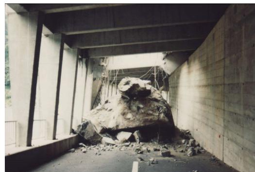
Fig. 3 Failed rockshed by large rockfall
