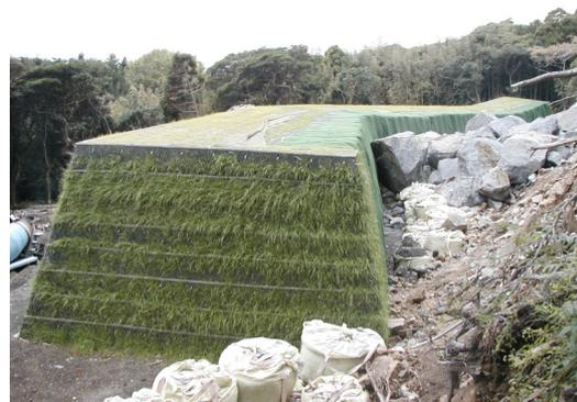
Fig. 2 Embankment for rockfalls
