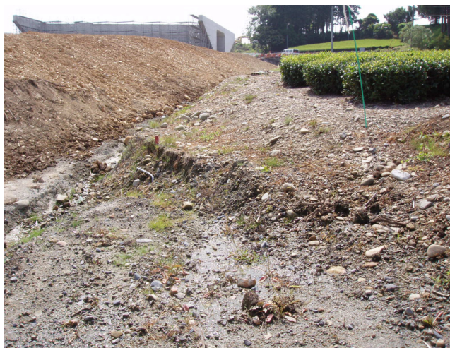
Photo 5 Earthworks Extended Close to Tea Plantation Field
