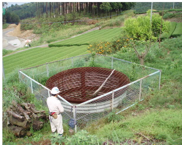
Photo 6 Drainage Well in Tea Plantation Field
