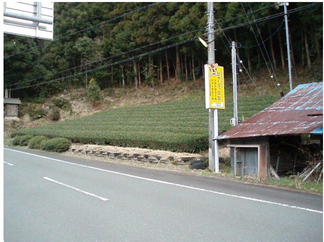
Photo 4 Tea Plantation Field in Past Landslide Site
