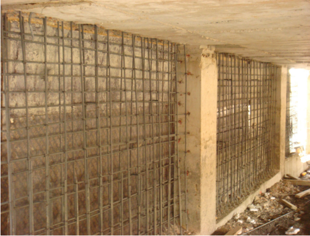
Figure 9. Installation of shear walls at expansion joints
