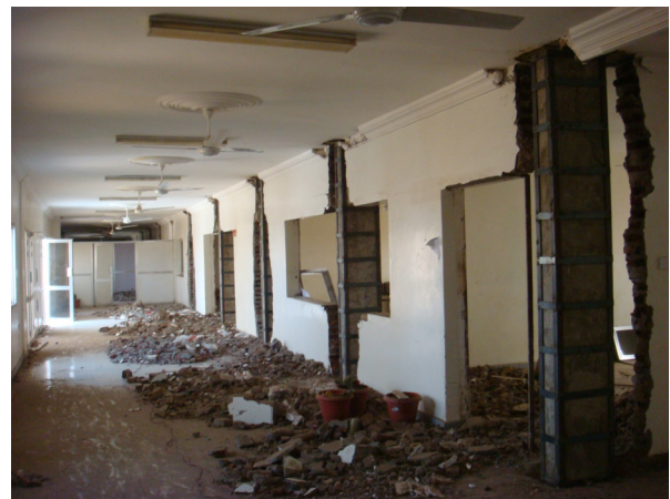
Figure 7. Metal jacking of second floor columns
