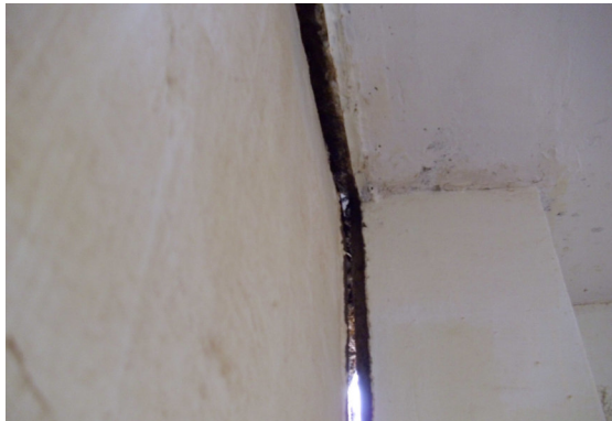
Figure 2. Opening at expansion joint.
