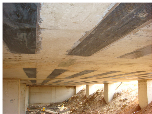
Figure 8. CFRP for basement cover slabs
