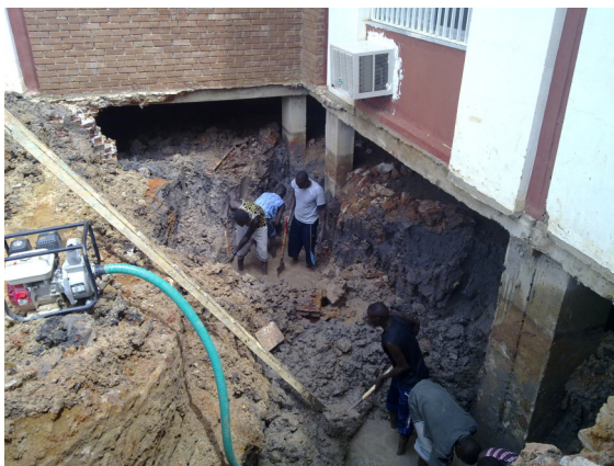
Figure 3. Dewatering during excavation.
