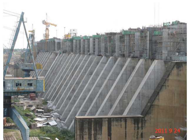
Fig. 2: Thickening and Strengthening of buttresses
