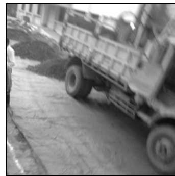
b) GSB spreading on Geotextile
