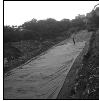
a) Geotextile above Murrum,
