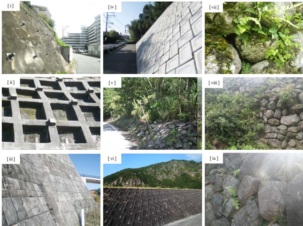
Fig. 1 Some examples of revetment techniques
