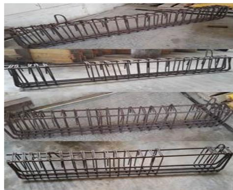
Fig.2. Details of the beam reinforcement.
