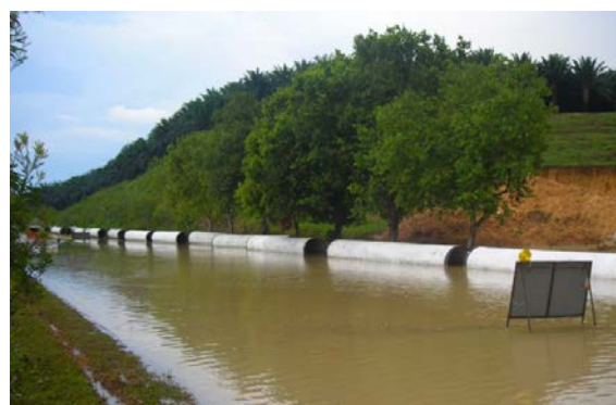
Fig.1: Typical road inundation during flash flood
