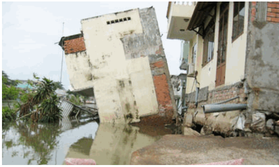
Fig. 2. The Building affected by riverbank failure
