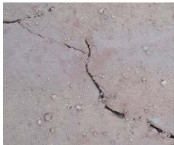
Fig. 2. Typical ground cracks reported in shale formation
