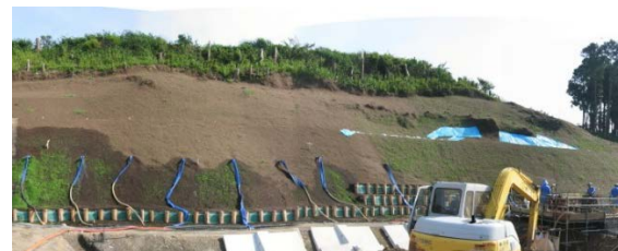
Photo 5 Horizontal Gravity Drains Installed on Temporary Cut Slope
