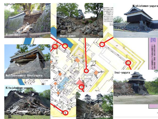
Fig.1 Several damages of Kumamoto Castle
