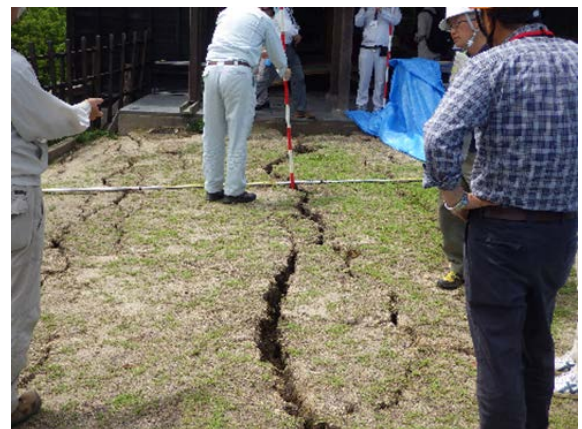
Fig.5 Cracking embankment
