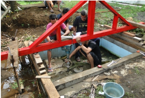
a. Photo of the still frame as bearing for field CBR
