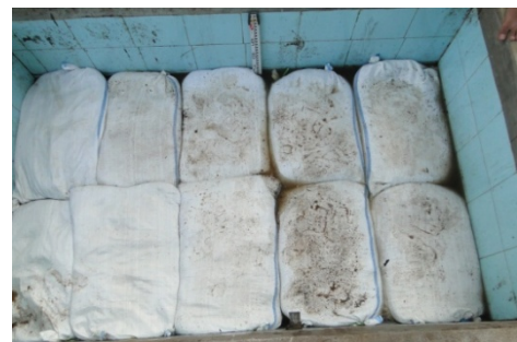
c. Soil bags placed on the bamboo pile
