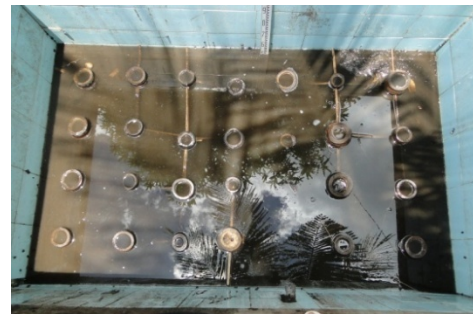
a. Bamboo pile installed in very soft soils
