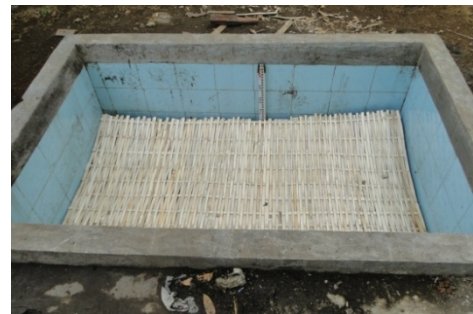
b. Geo-bamboo laid on bamboo piles
