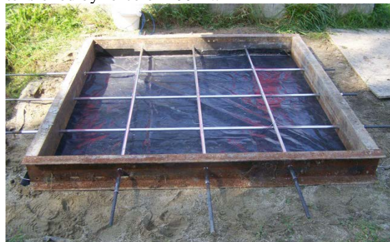
Fig.1 The steel formwork with ducts for prestressing bars
