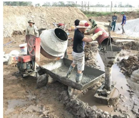
Fig. 3 CFG pile construction process
