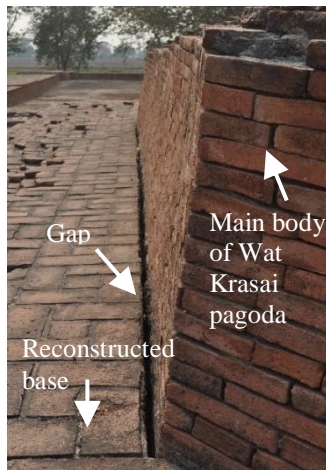
Fig. 4 The gap between the main body and the reconstructed base of the pagoda (Photograph taken on August 20, 2019)
