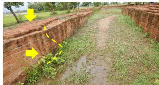
Fig. 3 Deformation of brick wall at Wat Krasai (Photograph taken on May 17, 2017)
