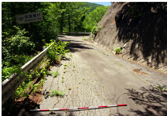
Fig. 5 Deterioration of road surface in the closed section of Gonbei Highway. Cracks, accumulated fallen leaves, and scattered invading weeds can be observed. Length of the red and white striped pole = 2 m.
