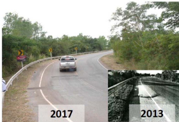
Fig. 14 Crack due to horizontal movement
