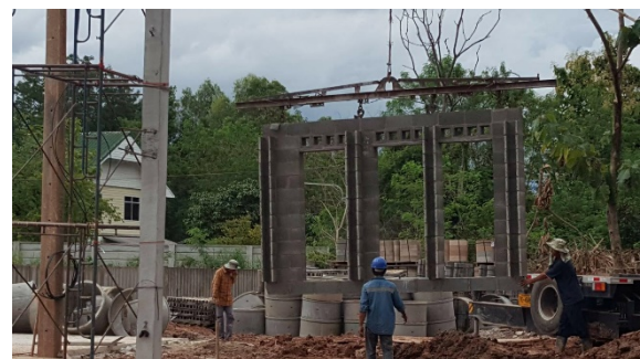
Fig.1 The rapid construction of wall using preformed concrete blocks
