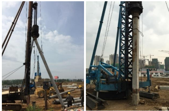
Fig. 2 (a) Open-end concrete pipe pile; (b) Precast square pile
