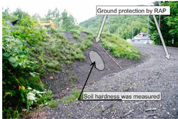
Fig.1 Ground protection by RAP
