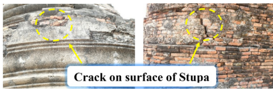
Fig.1 Example images of cracks on the surface of stupas visible in many locations around Wat Chai Wattanaram, a temple located in the historic province of Ayutthaya, Thailand.
