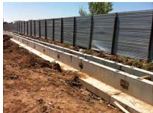
Fig. 7 The guide wall for diaphragm wall
