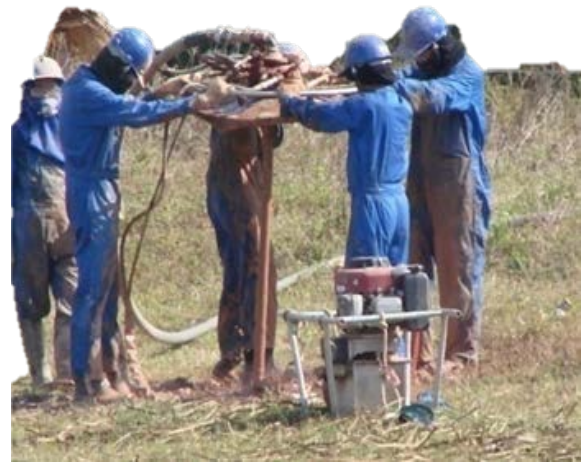
Fig. 3 Explosive installation
