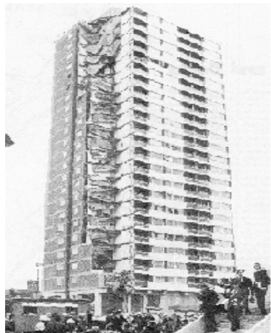
Fig.4 22 Storey tower-block in London partly collapsed 196 resulting in a zipper-type collapse (Designing Buildings Wiki)
