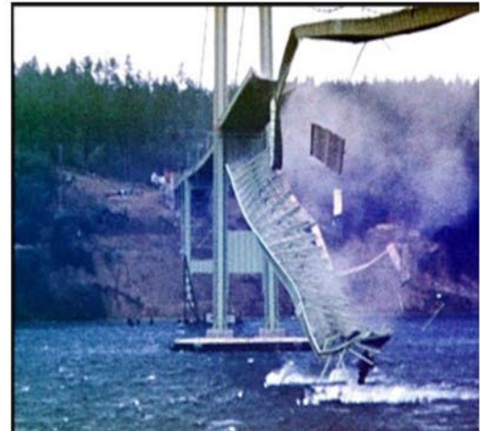
Fig.8 Tacoma Narrows suspension bridge in USA 1940 instability type progressive collapse (Wikimedia Commons)
