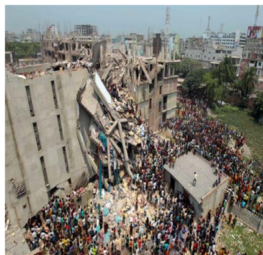
Fig.10 11 Storey Bangladesh building with several sections mixed type progressive collapses (National Geographic)
