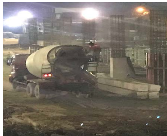
Fig.6 Distribution of Molen Truck for High Rise Building foundry with Fly Ash and Cement Slag
