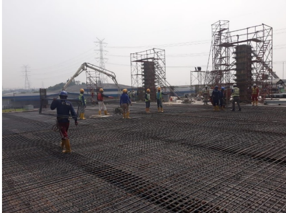
Fig.7 Floor and column concrete with concrete containing FA and cement slag
