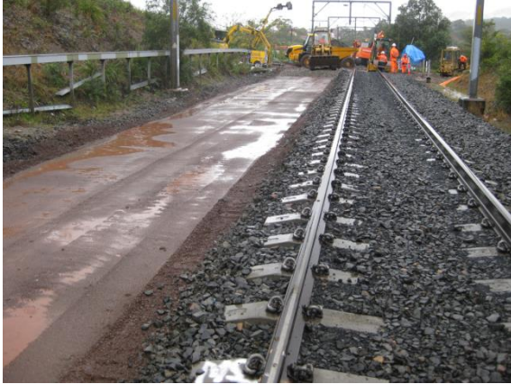
Fig. 1 Ballast and capping layer [2].
