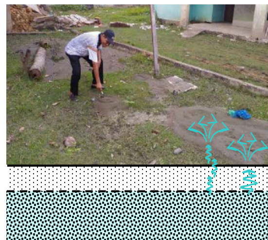
Fig. 5 Sand boiling due to Aceh earthquake 2016
