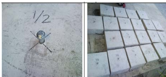
Fig. 2 Installed expansion anchor bolts in concrete bases
