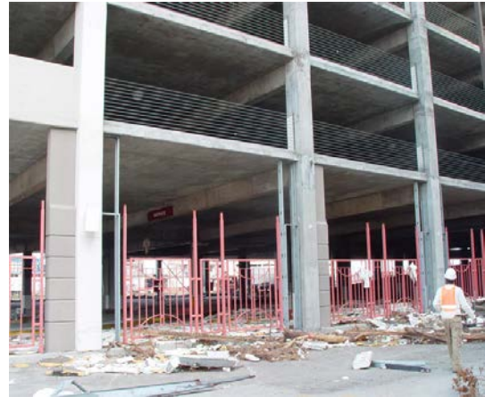
Fig.7 Cast in-place type structures where pre-preparation is critical (A4Architects.Nairobi 23 July 2014)
