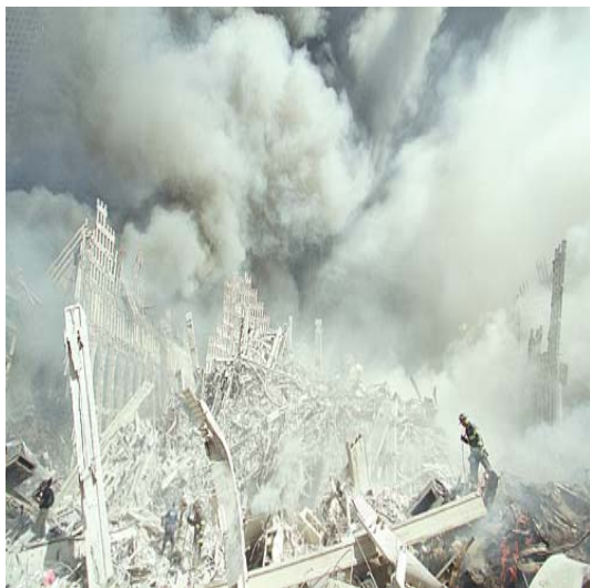
Fig.1 RC structures produce a cementitious dust cloud (9-11 Research.com 9 September 2015)
