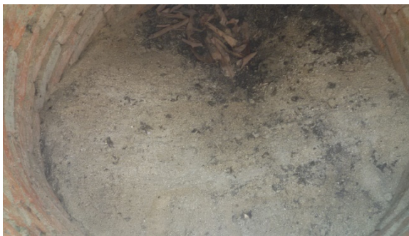
Fig. 8 Sand injected into wells of several houses replacing the groundwater.
